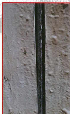
Placing of rods inside of the groove.
