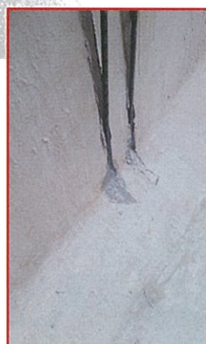
Anchoring of the rod into the slab using MAXFIX® E .
